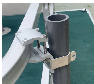
3. Top clamp, attached to PVC and top rail
